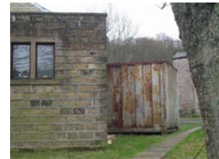
Container behind the church
