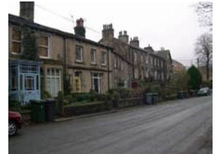
Carrs Road Terrace
