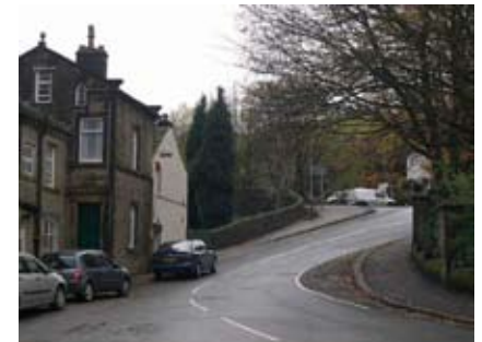
Floorscape and streetscape Towngate
