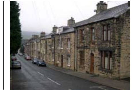
Brougham Road terracing
