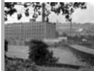
View of Titanic Mill from Lowestwood Lane
