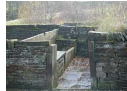
Stone troughs and dry stone walls
