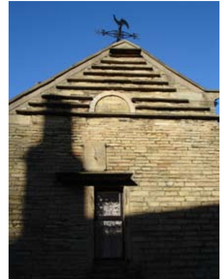
Distinct architectural features of Low House Farm
