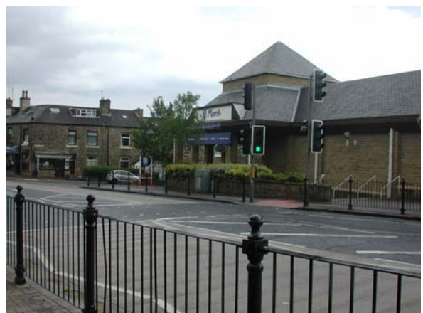
The Co-op, Westbourne Road
