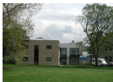
Primary care centre
