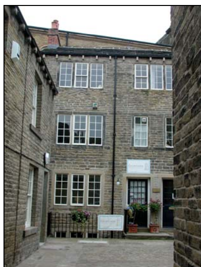
Above: Refurbishment of premises in Wormald's Yard
