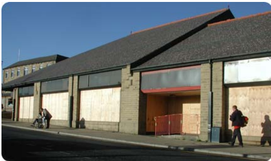
Vacant Kwik Save Store, South Street
