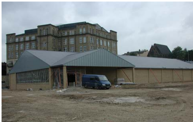
Lidl, Bradford Road, under construction
