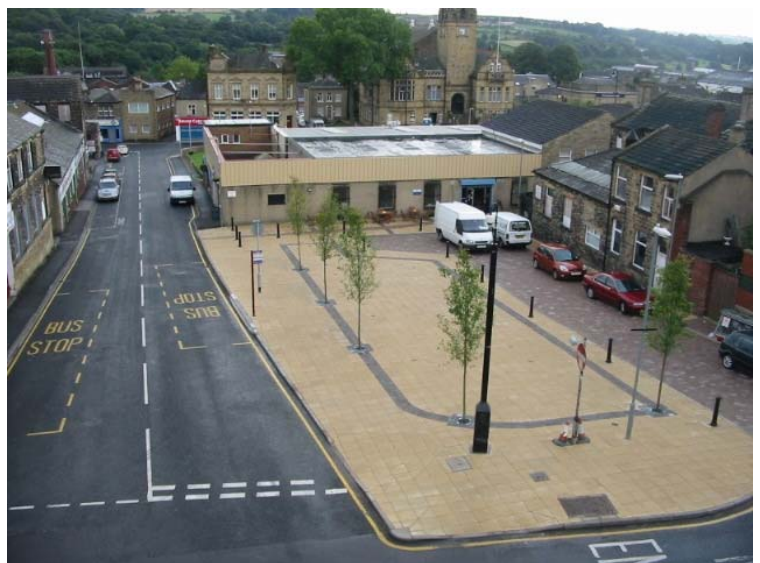
The refurbished Market Place
