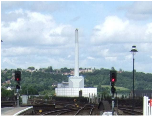
Figure 36 Huddersfield energy from waste plant in Kirklees (Source: © Copyright David Ward and licensed for reuse under this Creative Commons Licence, website accessed January 2011 www.geograph.org.uk/photo/489160 )
