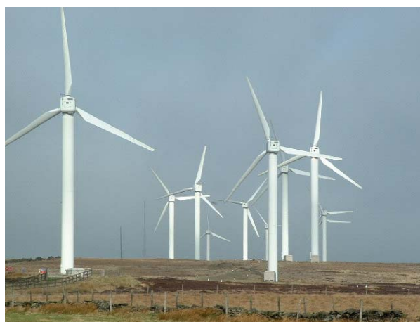
Figure 19 The 9 MW, 23 turbine, Ovenden Moor Wind Farm in Calderdale. This wind farm has been operational since 1993 and an application has been submitted to planning for repowering of the site with larger turbines. (Source: Nigel Homer, March 2005, retrieved from Wikimedia website, accessed November 2010)
