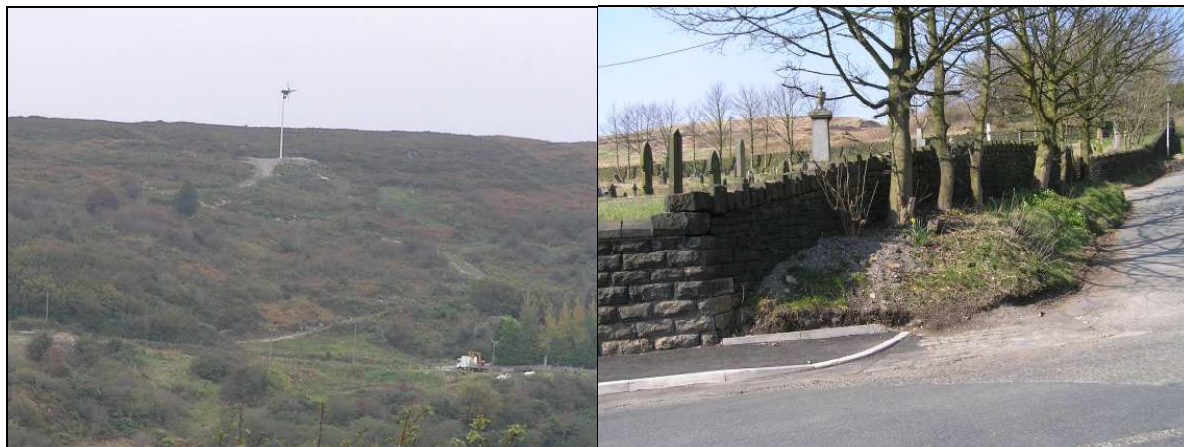
The access track and hardstanding for this small turbine on steep slopes (left) have scarred the landscape. Site access for large turbine components risks damage to traditional landscape elements (right) including walls and trees.
