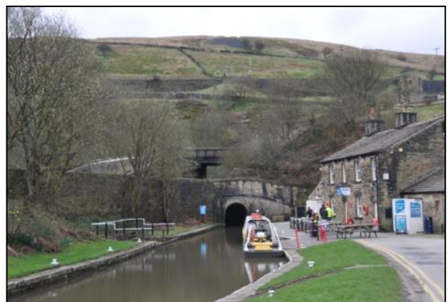
Figure 3.30: Standedge Canal tunnel
