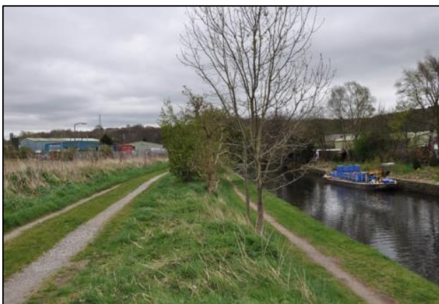
Figure 3.50: Bridge over canal from the towpath
