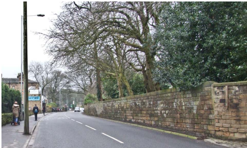
View south along Oxford Road near West Lane Fig 8
