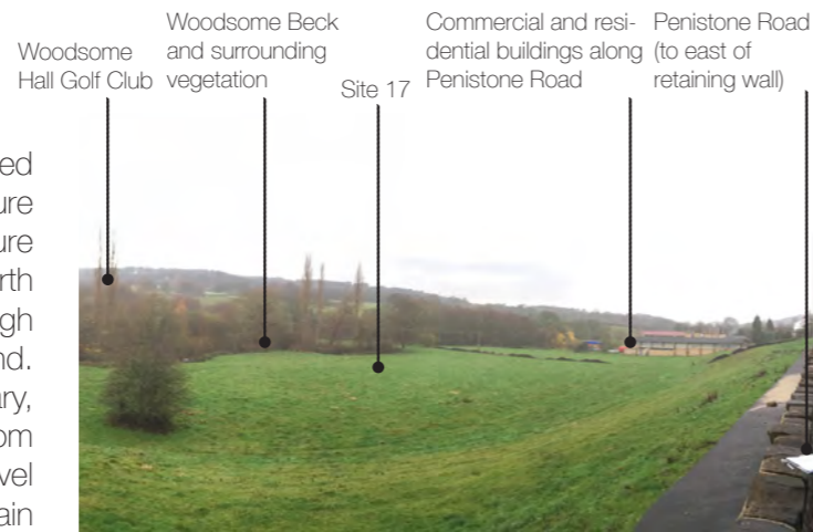
Site photograph looking to the north-west from Penistone Road at eastern edge of Site 17
