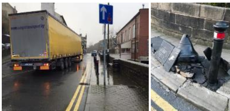
Figure 33 - Truck stuck on Hollowgate, Holmfirth & HGV damage to 'bell' protecting bridge on Hollowgate
