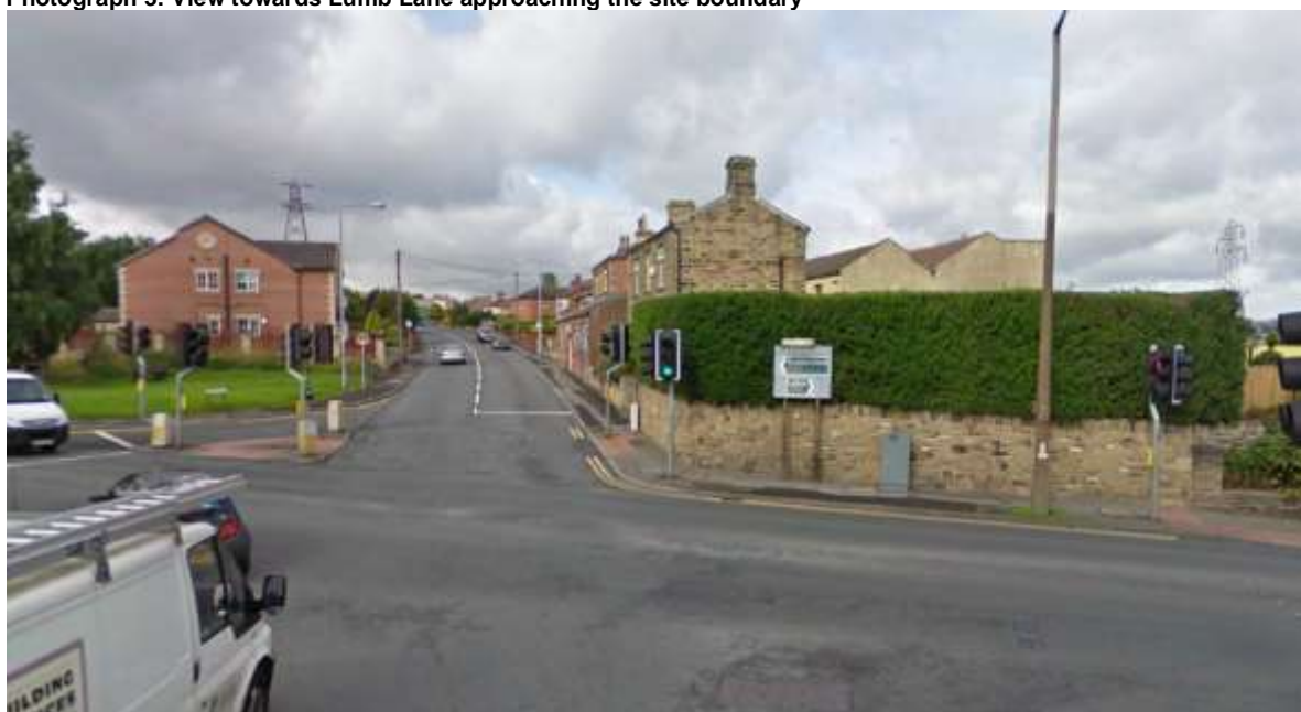
Photograph 3: View towards Lumb Lane approaching the site boundary
