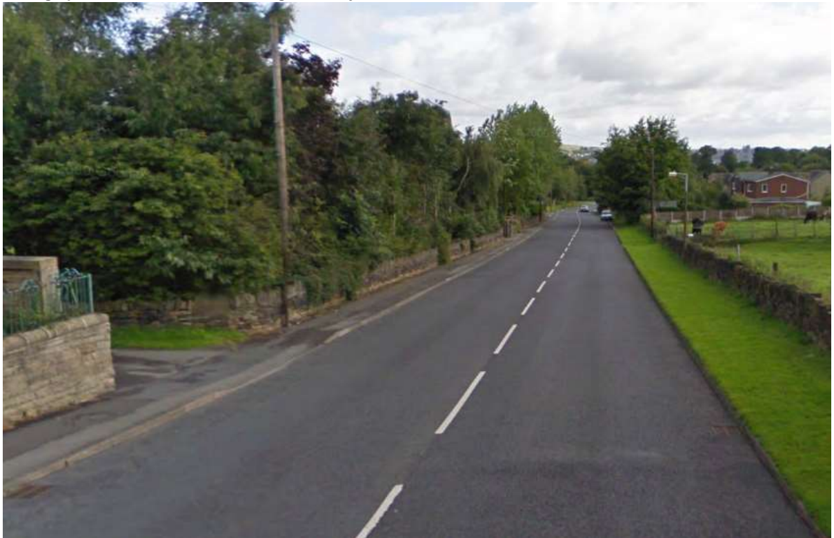
Photograph 5: Roberttown Lane, looking north adjacent to the site
