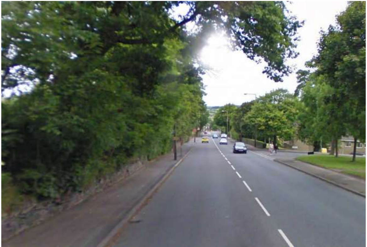
Photograph 7: A62 Huddersfield Road, looking north
