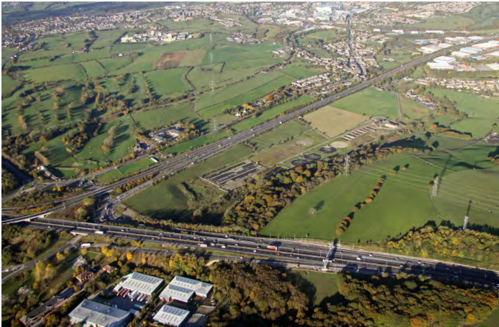
Figure 2: Aerial photograph of the site looking north-west towards Oakenshaw, Euroway and Low Moor
