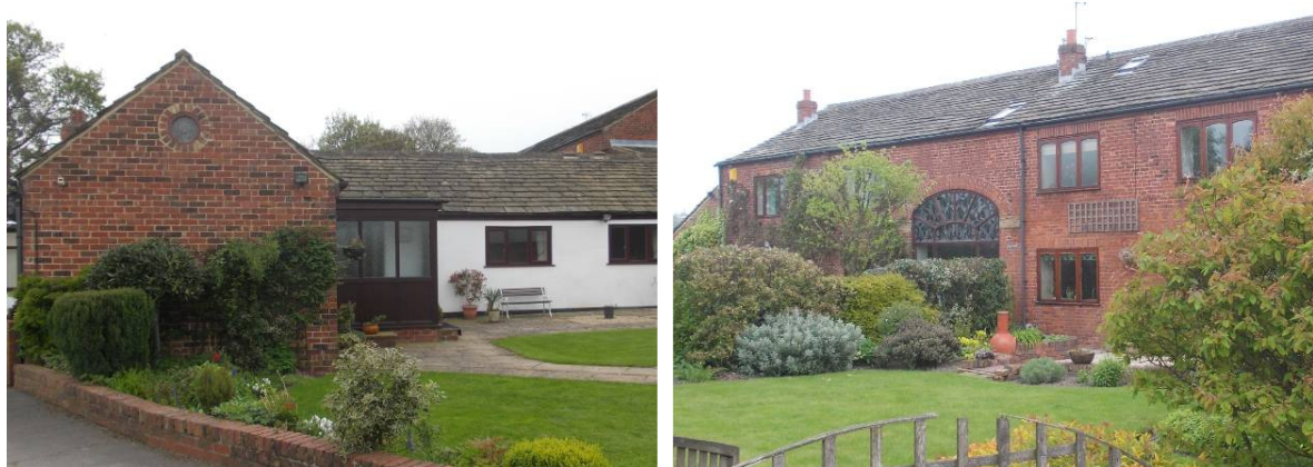
Figure 11 Views of the converted brick and render barn from the east (left) and north (right).
