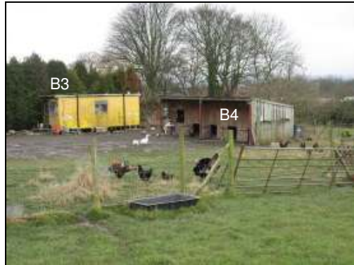
Buildings B3 and B4
