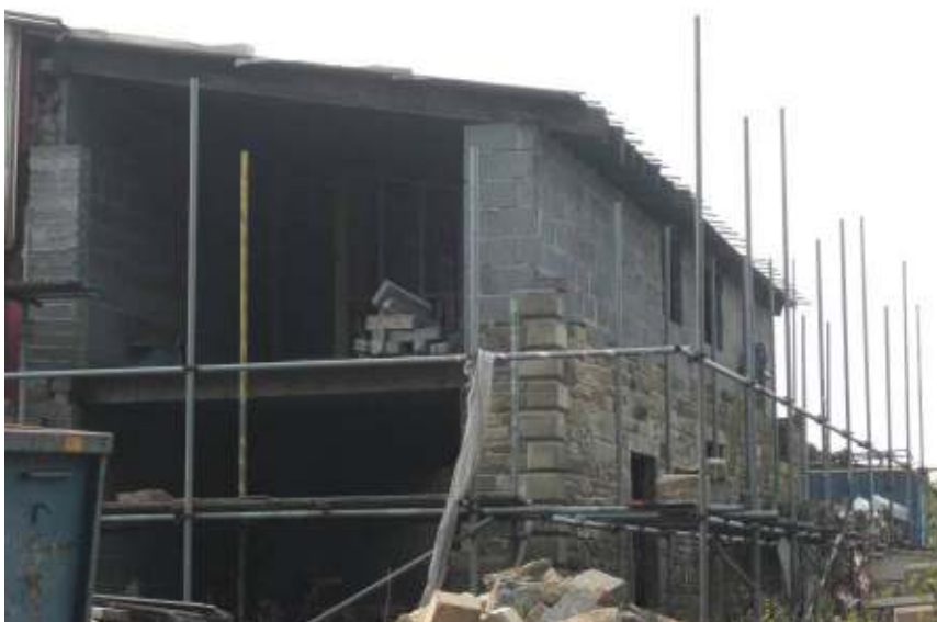
Photograph 5 showing building work being carried out at Thostle Nest Farm
