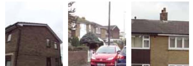
Roofing: concrete roof tiles in brown grey colour range predominates
