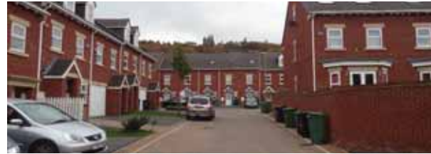
Olympia Gardens streetscape cul-de-sac showing of 2 and 2 1/2 story terrace dwellings with parking out front
