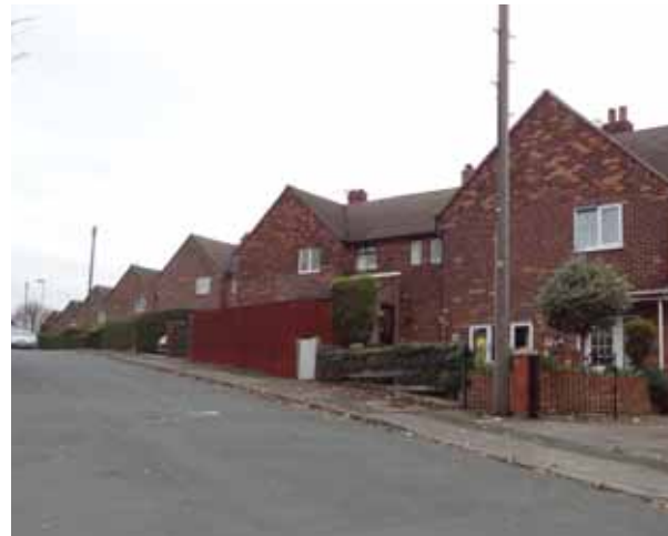
Dwelling set at an angle to the highway, creates visual continuity whilst minimising underbuild and retaining structures.
