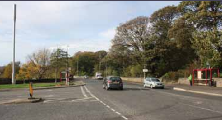
18. Huddersfield Road and Low Mill Lane Junction looking west
