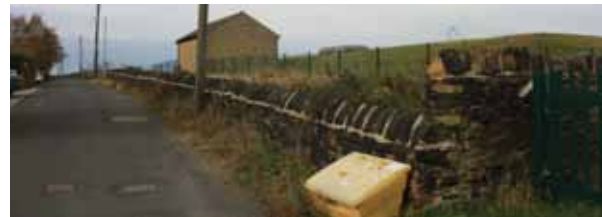
Retaining wall to Foxroyd Reservoirs
