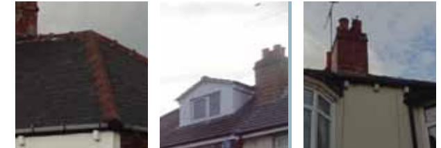
Roofing: Slate, clay or concrete roof tiles. Steeply pitched, hipped roof with deep eaves and central chimneys
