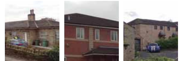
Roofing: natural stone slate is used for tiles and ridges with some concrete lookalike stone on the newer brick golf clubhouse
