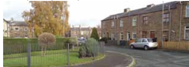
Terraced housing on Morton Grove constructed in natural stone, newer homes appear to be constructed in artificial stone for continuity.
