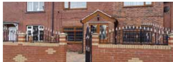
Large terraced units with walled boundaries and no driveway
