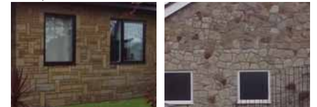
Walls : these are mainly buff brick or artificial and natural stone in a variety of coursing patterns.
