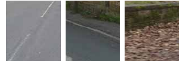
Surface Treatment: The surface treatment is made up of different paving with a variation of patterns helping to define different areas
