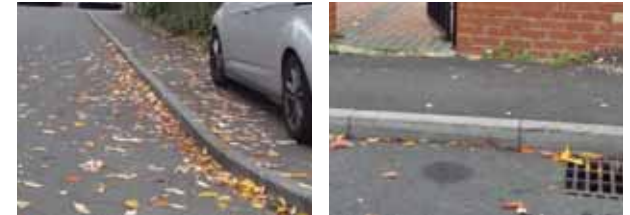
Surface Treatment: Both the pavements and the roads are made up of tarmac with concrete curb stones defining the pavement edge
