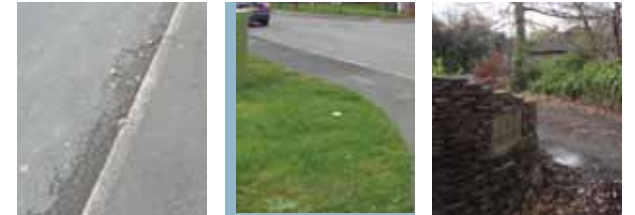
Surface Treatment: The pavements and the roads are made up of tarmac with some stone kerbs. Some drives are unsurfaced
