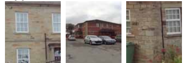
Walls: dressed natural stone is used on the older buildings with red brick and heavy stone coins to the golf club building
