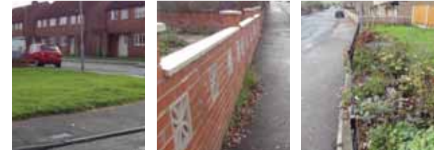
Boundary Treatment: Some walls are used in front of dwellings but grass or other vegetation is more widely used
