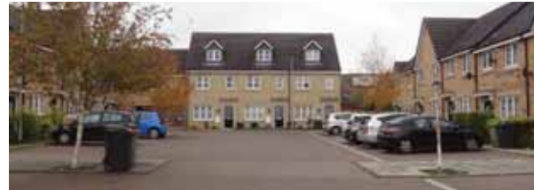
Providence Court southern cul-de-sac with a range of 2 and 2 1/2 story terrace dwellings with parking court for residents
