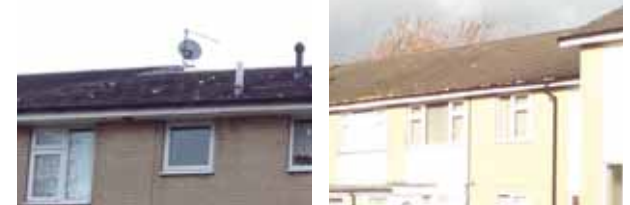
Roofing: Low pitched dual pitched roof with shallow eaves
