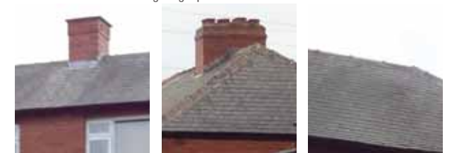
Roofing: Slate roofs pitched front to back with chimneys on the party wall. Deep eaves fit tight above window lintel
