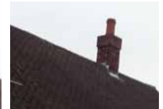
Roofing: Flat profile red/ brown tiles with shallow eaves.
