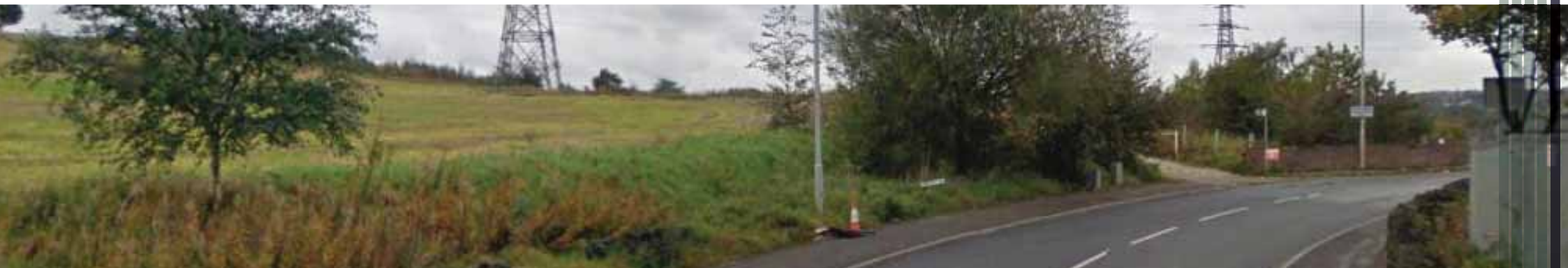
34. Ravensthorpe Road site access
