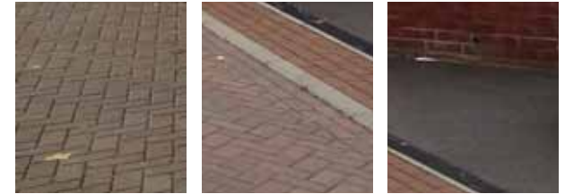
Surface Treatment: The surface treatment is made up of different paving with a variation of patterns helping to define different areas
