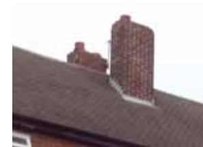
Roofing: Flat profile red/ brown tiles with shallow eaves.
