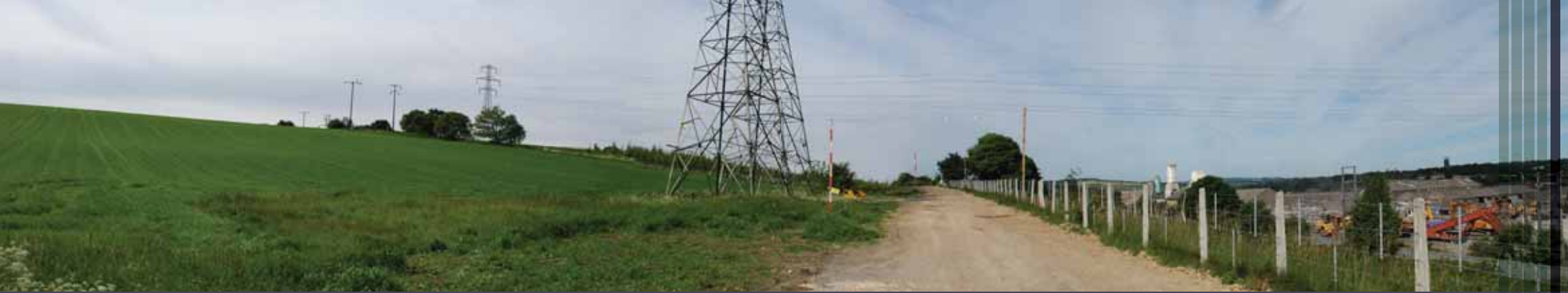
32. Footpath adjacent rail line
