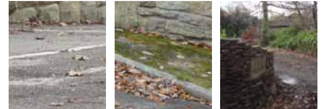
Surface Treatment: The pavements and the roads are made up of tarmac with some stone kerbs. Some drives are unsurfaced
