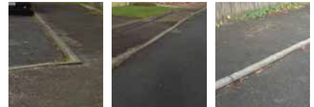
Surface Treatment: Both the pavements and the roads are made up of tarmac with curb stones defining the separation
