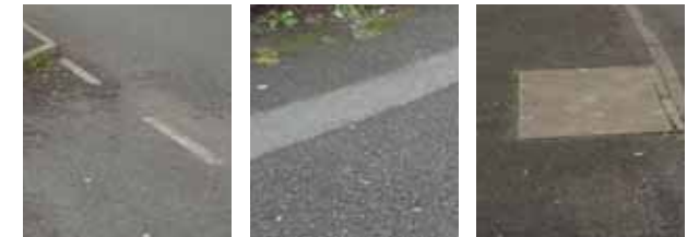
Surface Treatment: The area is made up of tarmac roads with evidence of roads being dug up and refilled
