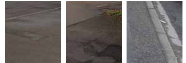
Surface Treatment: The area is made up of tarmac roads with concrete kerbs and edgings.
