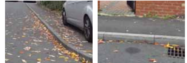
Surface Treatment: Both the pavements and the roads are made up of tarmac with curb stones defining the separation
