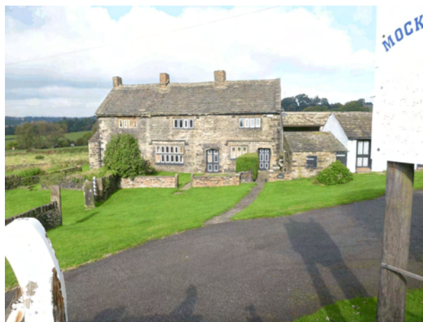
Plate 26 Mock Hall, looking northwest
