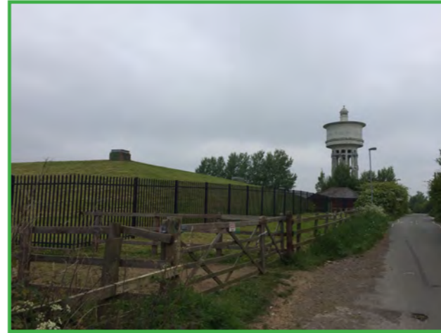
Photograph 12 - View from Chidswell Lane on the approach to Gawthorpe Reservoir and Water Tower
