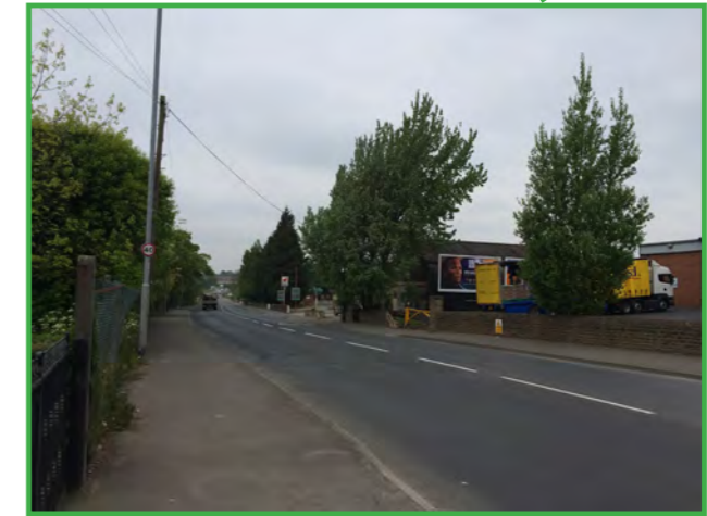
Photograph 19 - View along Owl Lane towards Site - a belt of coniferous trees limits view of Site
