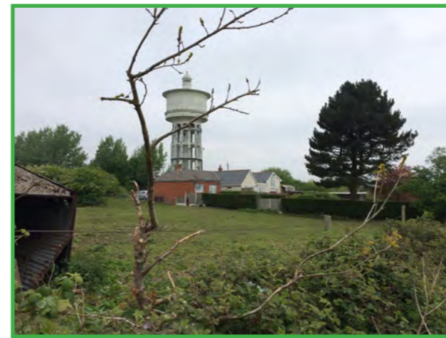
Photograph 3 - View towards Chidswell Lane and properties at Chidswell Dene
