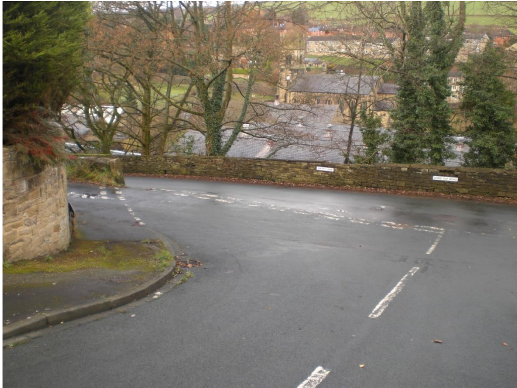
Photo 7 Taken 2.4metres from the Bankfield Drive junction and showing the wall which obstructs the view down Smithy Lane, second on left. There is a drop of approx. 30 metres beyond the wall shown along Dobb Top Road.
