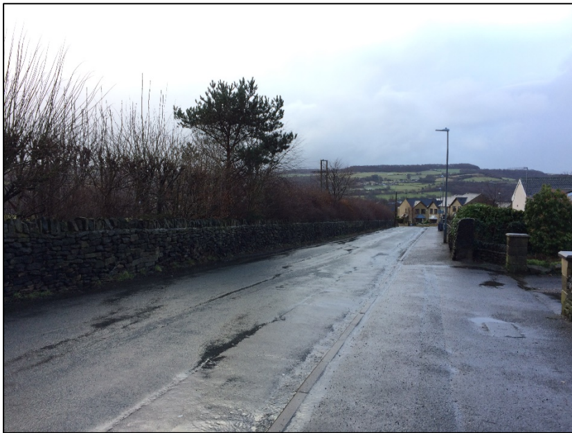
Plate 3: View north-east along southern site boundary on Scotgate Road
