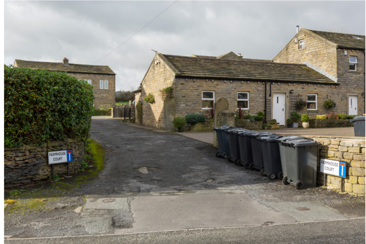
11. GLIMPSED VIEW THROUGH LISTED BUILDINGS AT FARMHOUSE COURT
