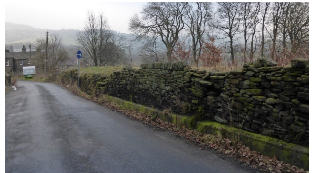
Figure 9 - View west along Pell Lane
