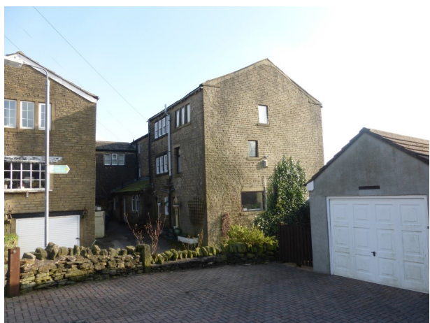
Figure 5 - View of the setting to the asset
