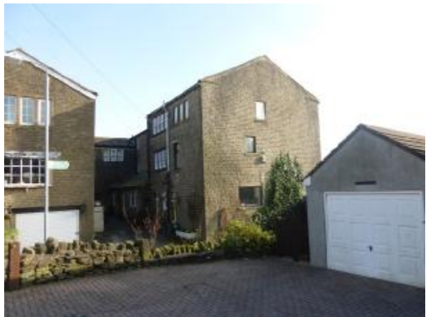
Figure 5 - View of the setting to the asset
