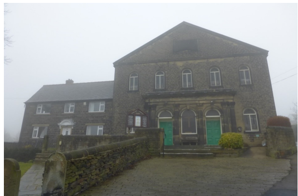
Figure 3 - South facing elevation
