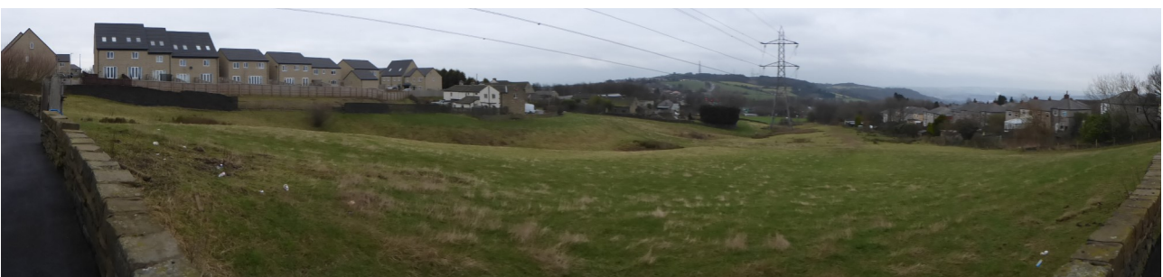
Figure 4- Panoramic photograph of the site from Weather Hill Road
