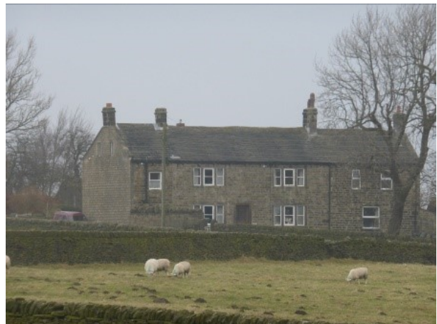
Figure 3 - Sandy Gate, south-east elevation
