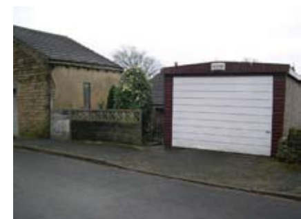
Garages, Verity Street
