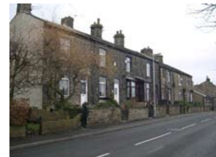
Terrace, North side of South View Road
