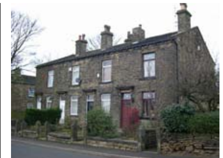
South View Road
