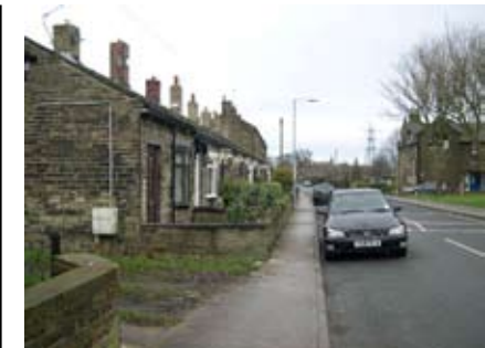
Low terrace of cottages, South View Road
