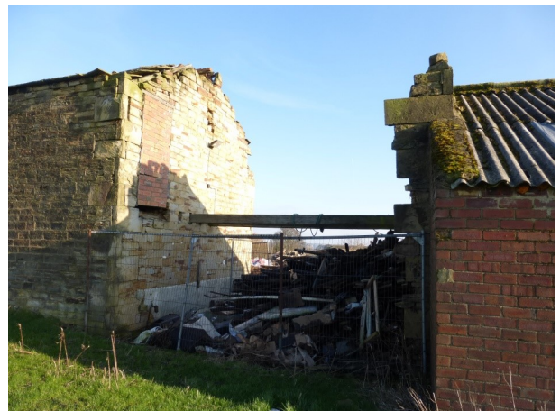
Figure 4 - View of the south elevation to Thornbush Farm from the footpath
