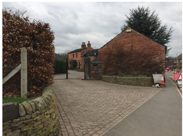
Figure 8 - View From Hagg Lane
