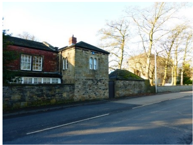
Figure 12 - view of The Red House from the east
