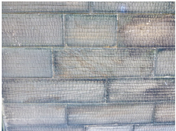
Figure 7 - The stone tooling
