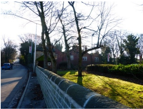
Figure 11 - view of The Red House from the north
