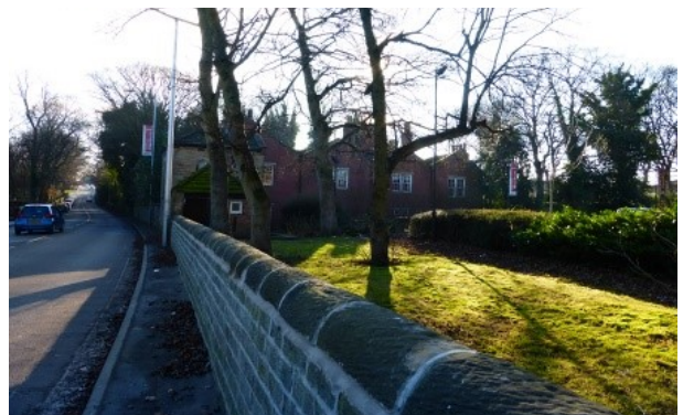
Figure 2 - view of The Red House from the north
