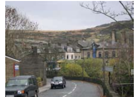
Roofscape from Station Road
