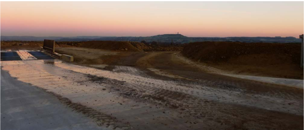
Figure 3: Photograph taken from the entrance to the site with Castle Hill in the background
