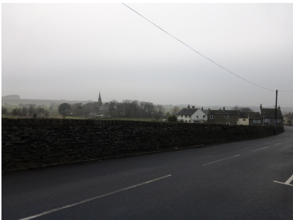
Figure 12: View of the boundary wall to area 2
