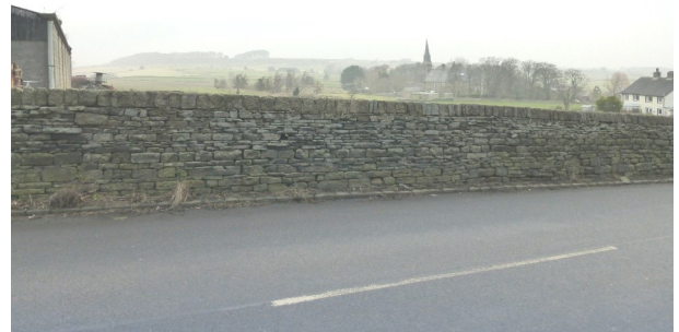
Figure 11: view of the boundary wall to Area 2
