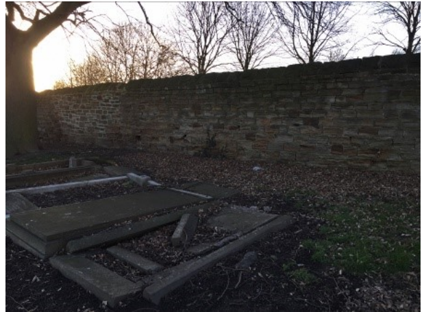
Figure 6 - View of the boundary wall
