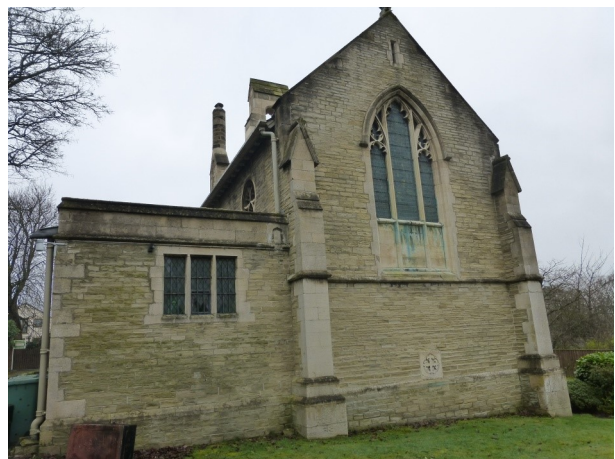
Figure 4 - View of the east elevation
