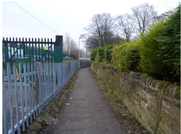
Figure 3 - View of the footpath adjacent to the historic asset
