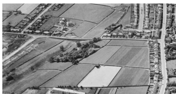
Figure 4 - View of the asset from 1937
