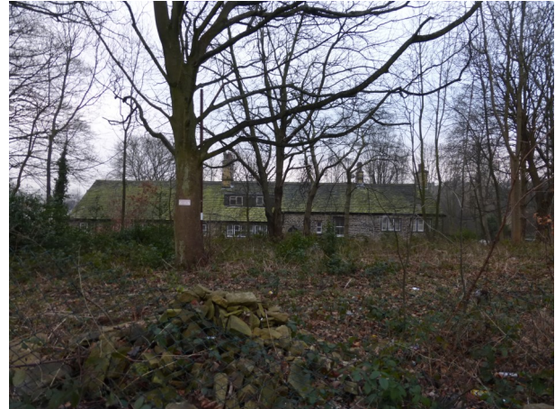
Figure 2 - View of the asset from the footpath
