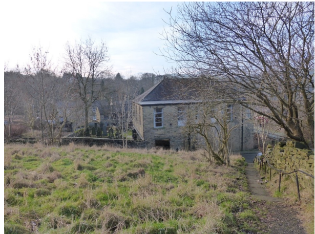
Figure 5 - View of the east elevation of the Providence Baptist Chapel
