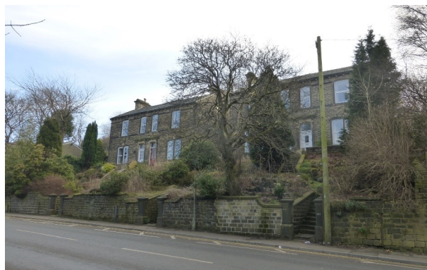
Figure 9 - View of the adjacent semi-detached dwellings
