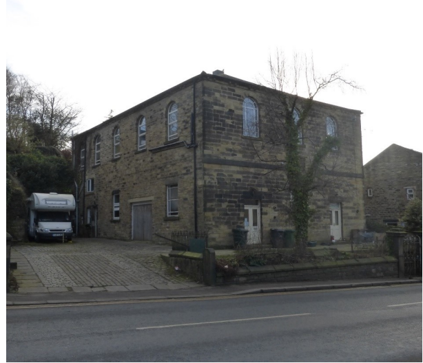
Figure 8 - View of the north elevation to the former chapel
