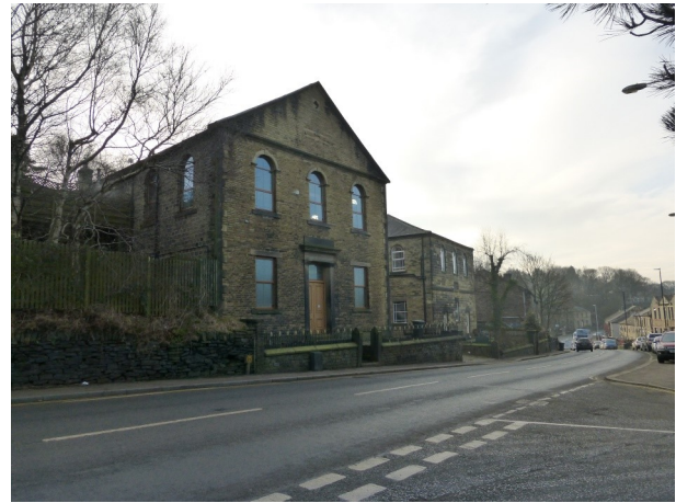
Figure 3 - View of the former Methodist Chapel and School Room
