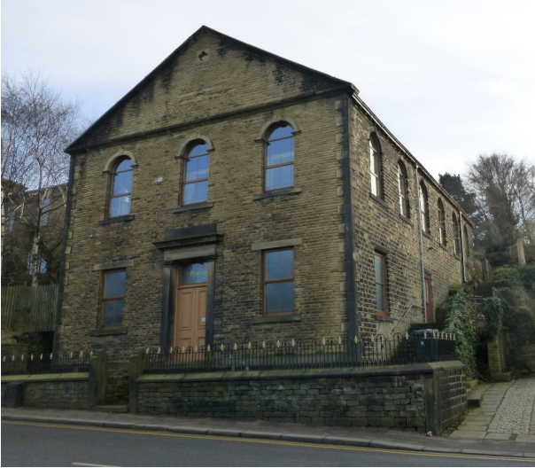
Figure 7 - View of the north elevation to the former school
