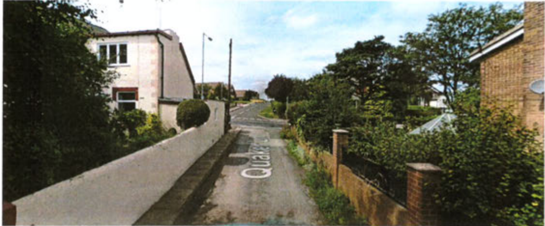
(Photo 2: Existing access along Quaker Lane, onto Hightown Road)
