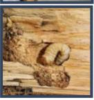
It is important to identify the cause of damp. The most common reasons are lack of ventilation, high external ground levels, leaking roofs, cement renders and concrete floor. These all encourage the build-up of moisture in the fabric of the building making it damp and providing the conditions for beetle and fungal
