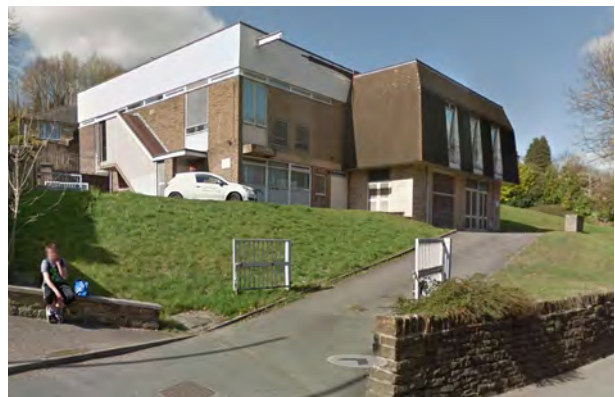
The telephone exchange is located at the approach to the town centre. This could be redeveloped to provide much needed accommodation in the centre of Holmfirth.
