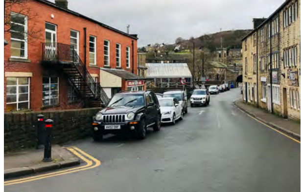
Holme Mill occupies a prominent corner in the town centre and could come forward for redevelopment in the future.
