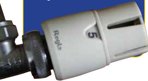
This is where the TRV is connected to the radiator and where hot water flows into the radiator itself.
