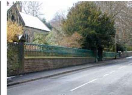
Gatepiers and railings
