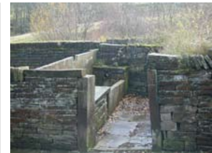
Stone troughs and dry stone walls
