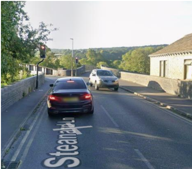
Figure 4 - Traffic signal control to ensure single lane flow
