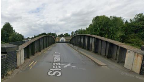
Figure 3 - existing bridge showing bollards in footway to prevent vehicle overrun
