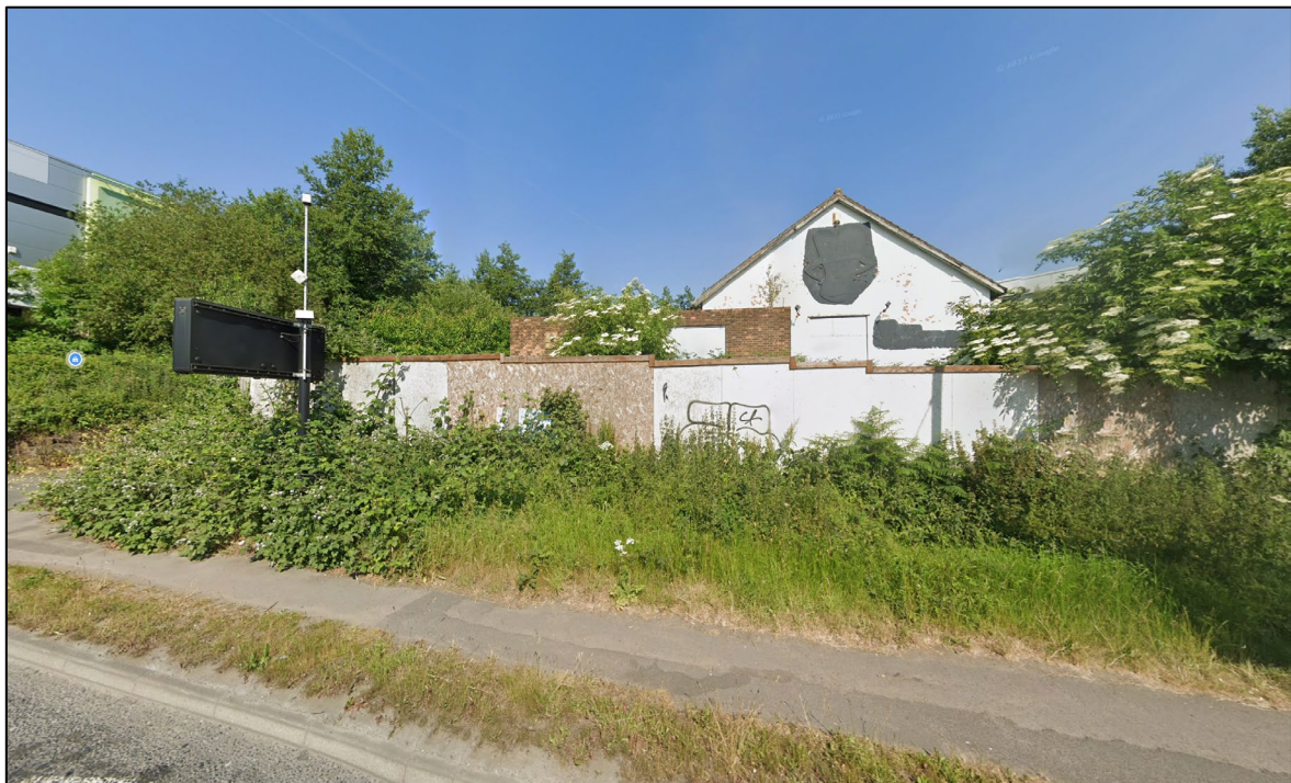
Figure 3.4. Existing Site [Viewed from Gelderd Road]
