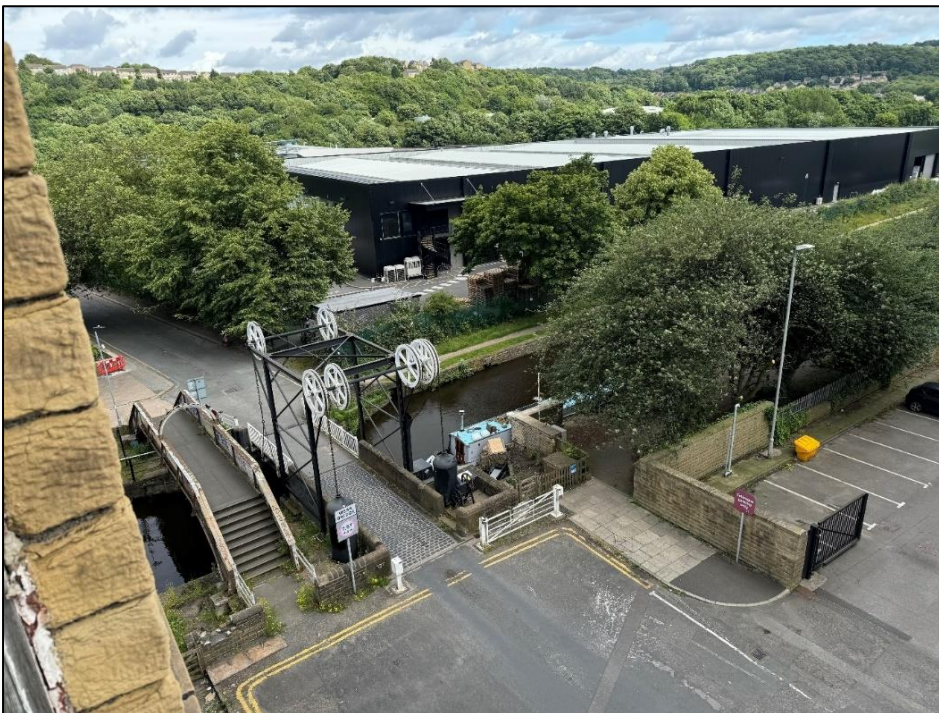
Figure 16: Industrial development approved and built within the immediate setting of the designated heritage assets at Turnbridge Mills with the Scheduled bridge shown in the foreground (application number 2015/92014)
