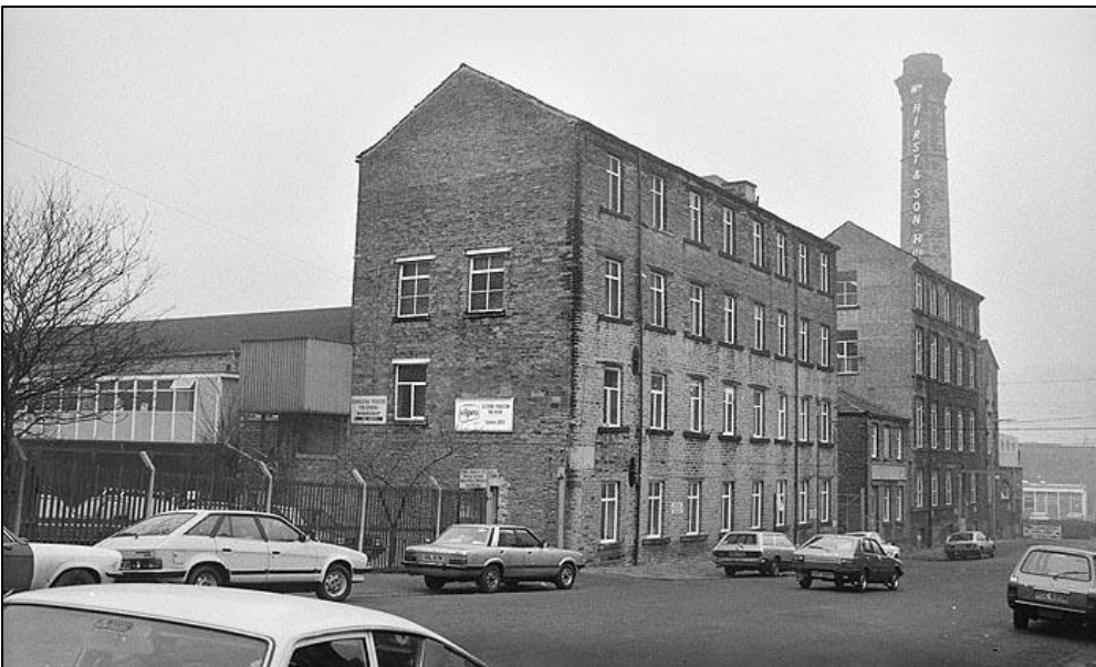
Figure 9: The original Building F before its replacement soon after this photograph was taken by the current two-storey building. Note also part of Buildings E, D, C and M as they appeared in the late 1980s (Historic England Archive reference mf078_q_34)
