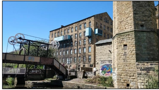
Figure 14: Grade II listed Building H to rear of bridge
